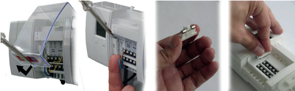
Fig. 49: Replacing the fuse
